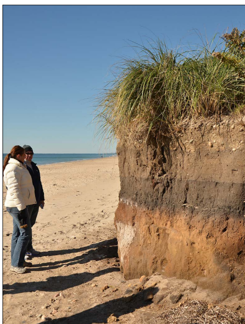
Erosion at Matunuck Beach after Superstorm Sandy. Photo Credit: Rhode Island Sea Grant
